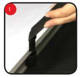
Insert and secure 1 pole arm into the bottom rail extrusion.
